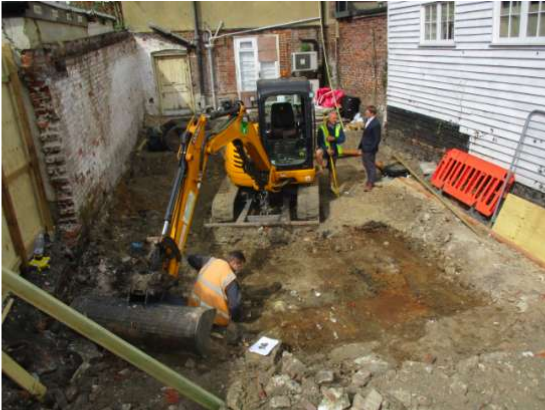
Plate 4. Clearing the site
