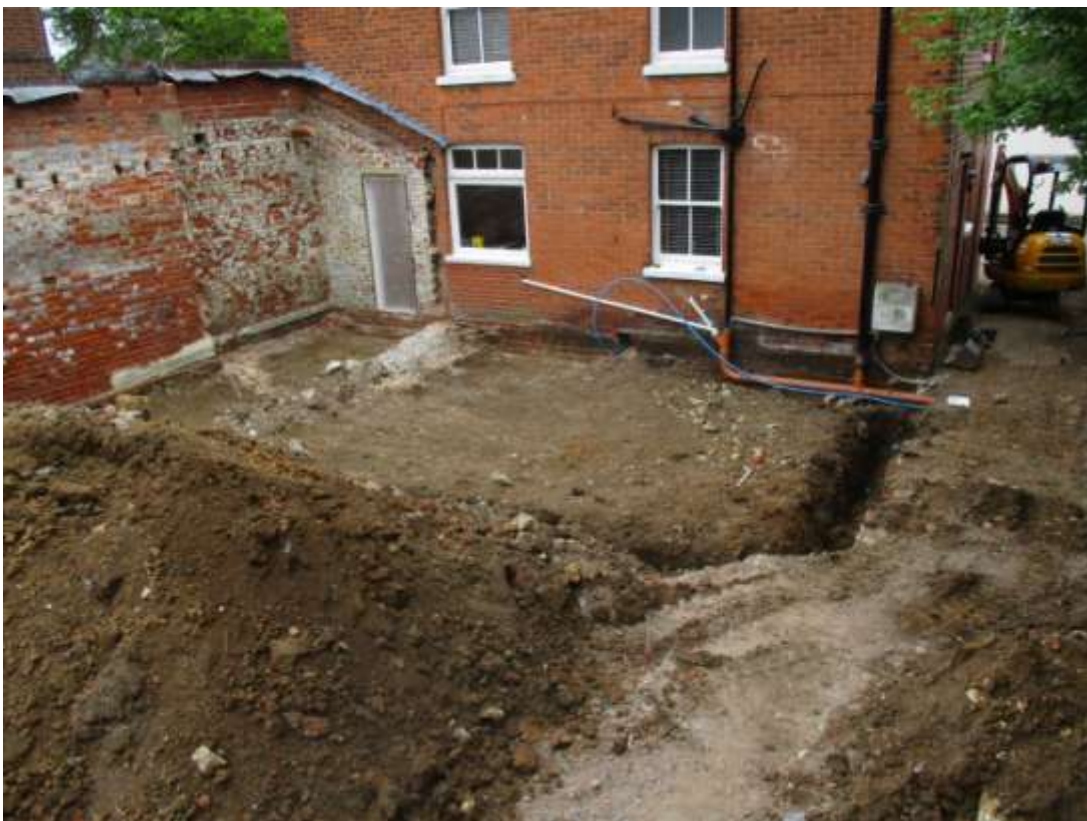
Plate 5. View of trenching
