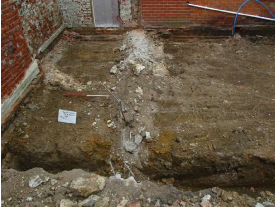
Plate 6. Close up of trenching
