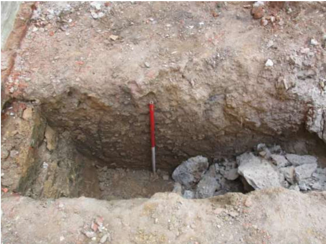
Plate 9. Section of foundation trench
